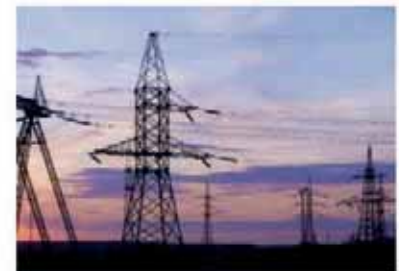
High Voltage Lines Management System
